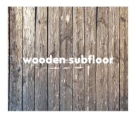
Check the floor for insect infestations. Make sure the subfloor is levelled and screw down any loose sections firmly. Wooden subfloors should always have access to air and should be ventilated at the edges. If there is any moisture in the wood-based subfloor or there is no proper moisture barrier below the wood-based subfloor, it must be removed first.
