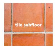
Check the subfloor for moisture problems. The joints of the new floor covering should never be aligned with the underlying tile joints. It is not necessary to fill the grouts of a subfloor comprised of ceramic tiles with joints when these do not exceed 5 mm in width. Bear in mind that some ceramic tiles may show rising edges/corners although the main level may be correct. These parts may telegraph through the floor covering in the future.
