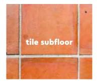
SPIRIT Gluedown can only be installed on top of firmly levelled subfloor for all gaps between ceramic tiles will telegraph through. Installation directly on unlevelled top of ceramic tiles is not recommended!
