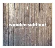
spirit Gluedown cannot be installed on most wooden substrates without special preparation. Either specific levelling compounds must be used, or the wood subfloor must be covered with special layers, e.g. plywood panels. These panels must be firmly attached to each other/the wood substrate and/or be glued or fixed. If there is moisture in the wood-based subfloor or there is no proper moisture barrier below the wood-based subfloor, it has to be removed first.
